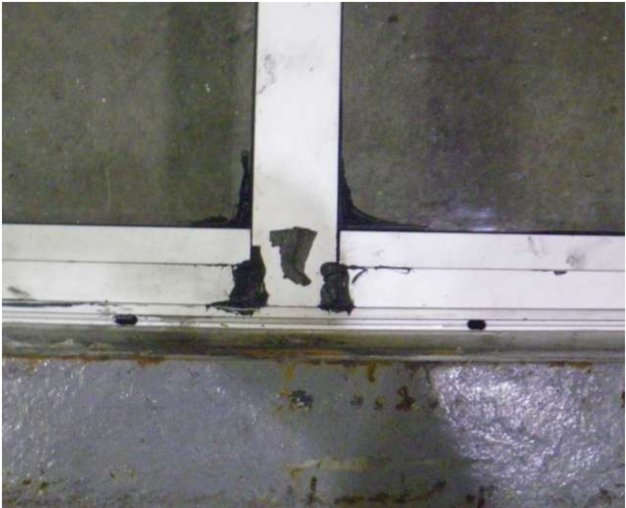
Photograph #1 Sealant At Glazing Gasket Joints
